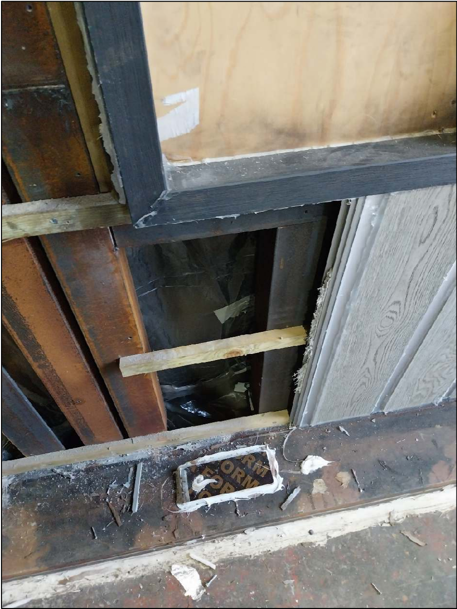
PLANKS REMOVED FROM SUPPORT FRAME
